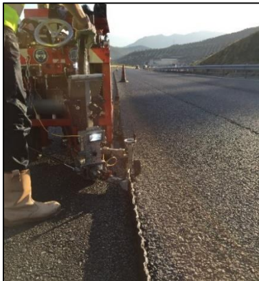
Fig. 2: Joint installation using the TOKOMAT® process
