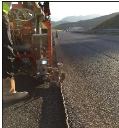
Fig. 2: Joint installation using the TOKOMAT® process
